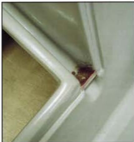
G10 epoxy board baffles installed in drainage gutter exits. Note location of weep hole above the baffle.
